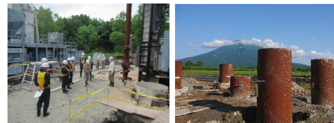
Experimental construction of soil cement piles for steel pipes for the Hokkaido Shinkansen
