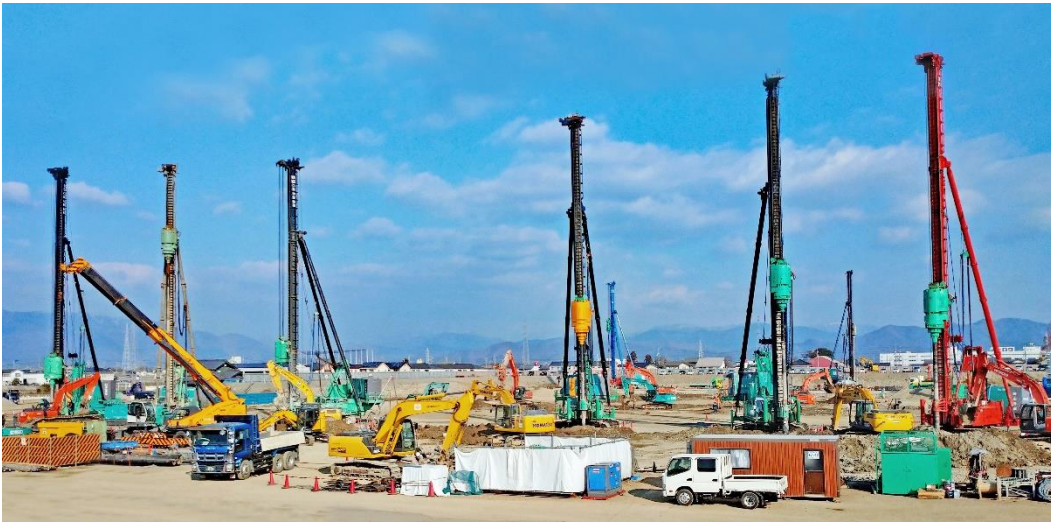
Construction of a new factory for an electronic component manufacturer (Ono Town, Gifu Prefecture) (performed between December 2022 and March 2023 using the Tenocolumn method)
